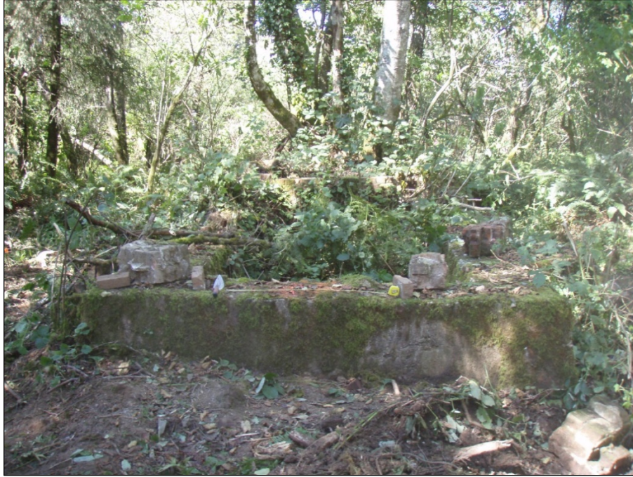
Figure 4. Overview of the foundation with portion of brick wall visible in the background; view to the north.
