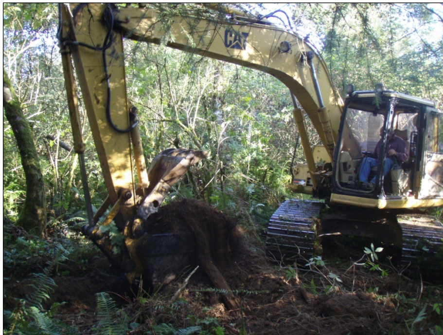
Figure 3. Overview of the Sadri-East Parcel environmental trenching; view to the northeast.
