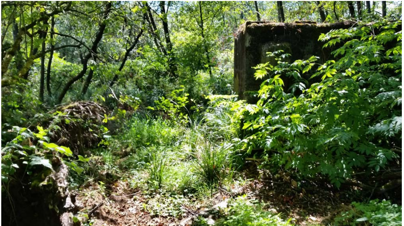
PHOTO 8: Large concrete foundation on West Mill..
