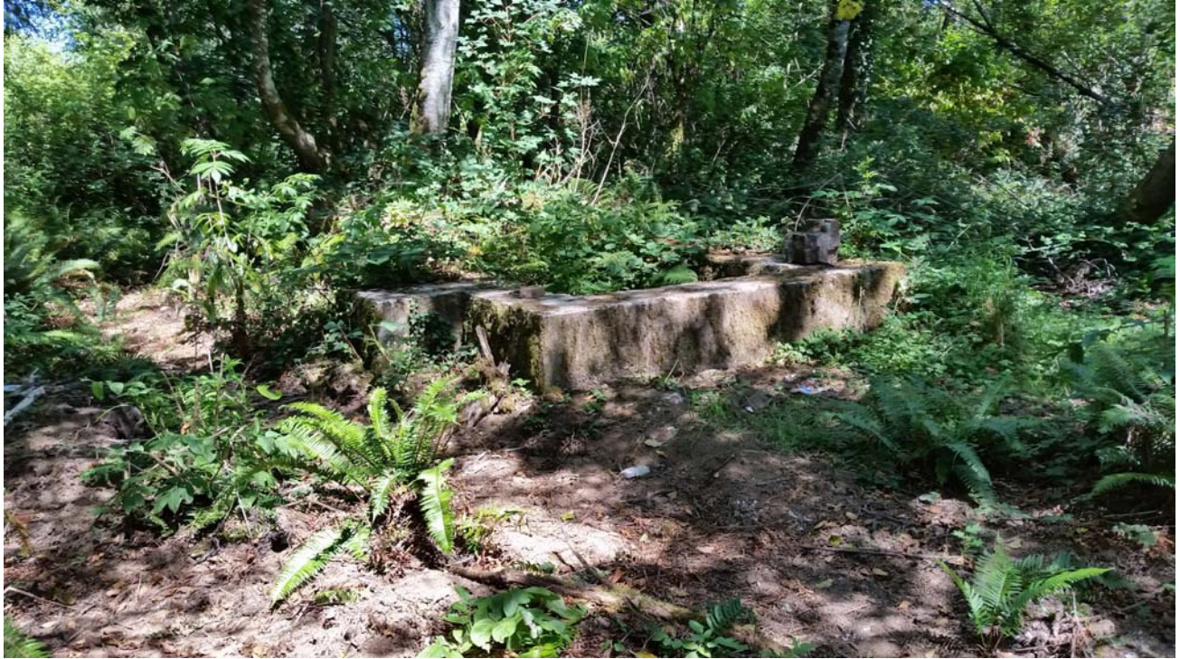
PHOTO 3: Concrete structure in former location of machine shop and boiler (former East Mill).
