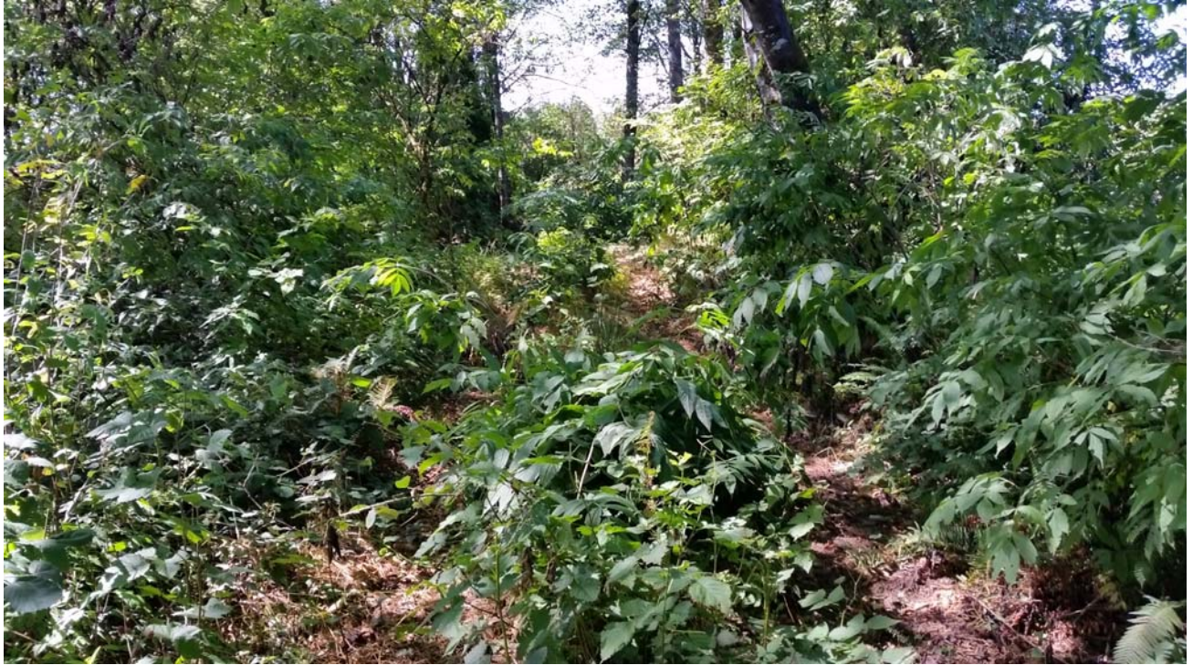
PHOTO 7: Typical view of overgrown foot trail on top of levee.
