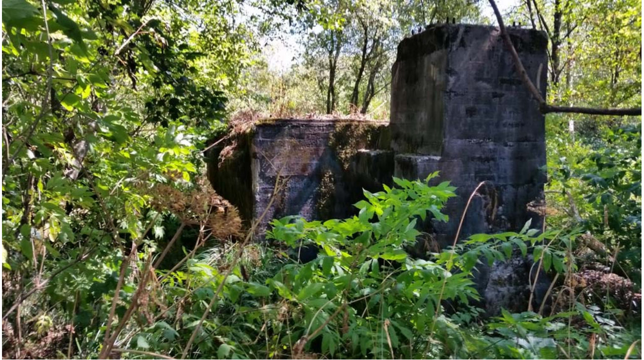
PHOTO 9: Closeup view of concrete foundation on West Mill.
