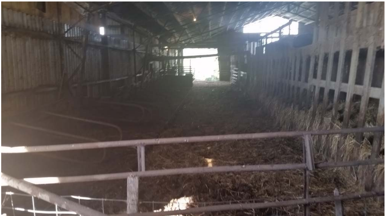
PHOTO 8: Interior of loading shed.
