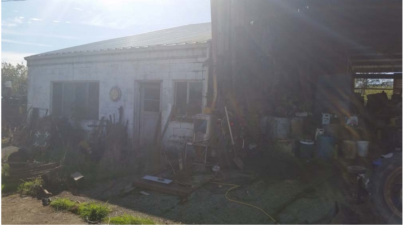
PHOTO 3: Items stored outside near east breezeway between former milking parlor and loading shed.
