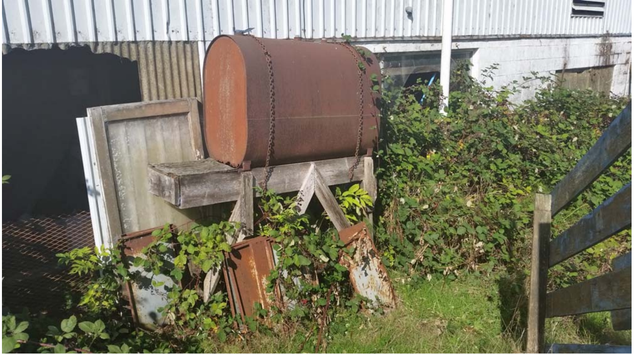
PHOTO 15: Above-ground oil tank (empty) on east side of milking parlor.
