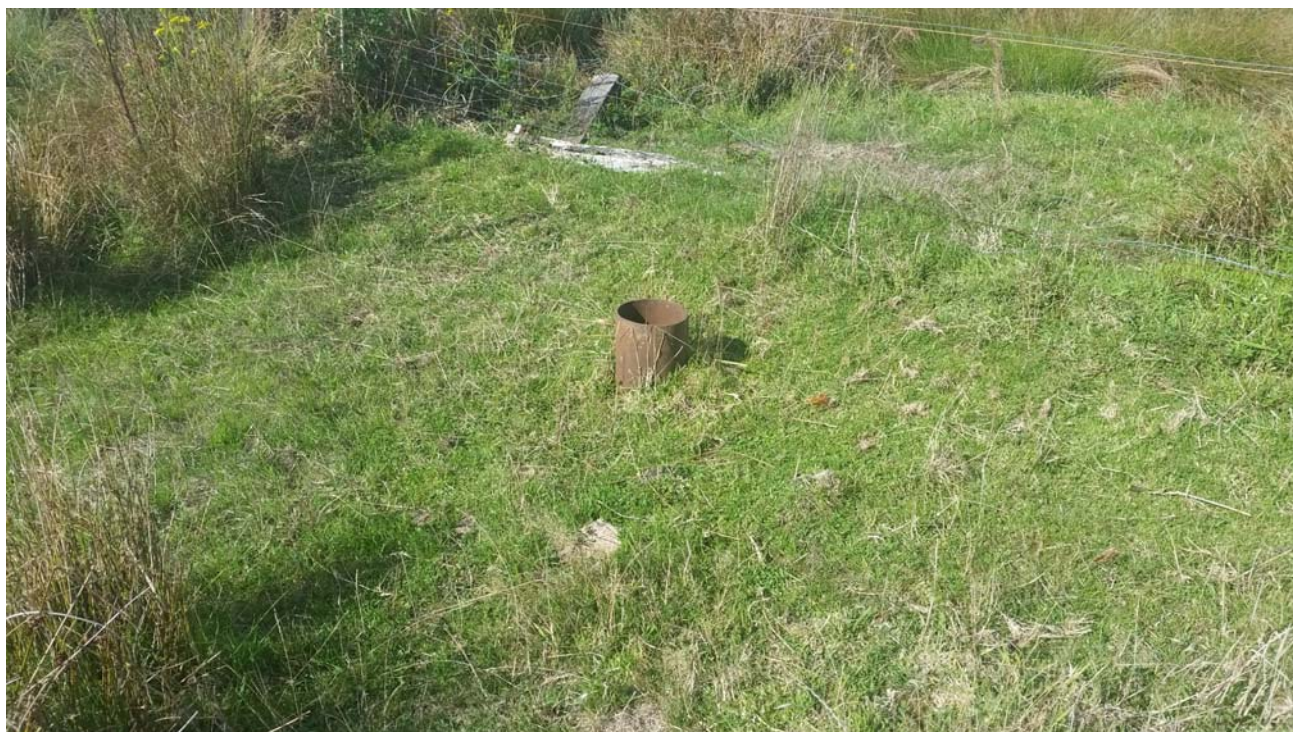
PHOTO 18: Steel casing for water well on tax lot 600, south of Goodspeed Road.
