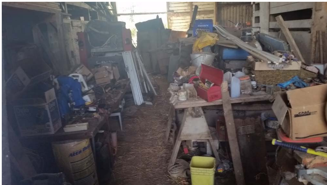
PHOTO 5: East breezeway between loafing shed and milking parlor. Floor is concrete.
