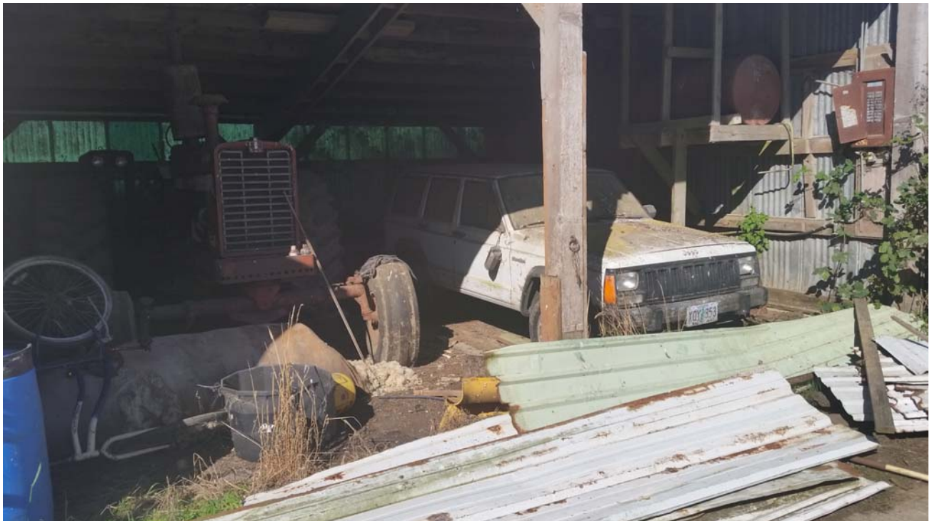
PHOTO 16: Machine shed. Note empty oil tank mounted on rack attached to north wall.
