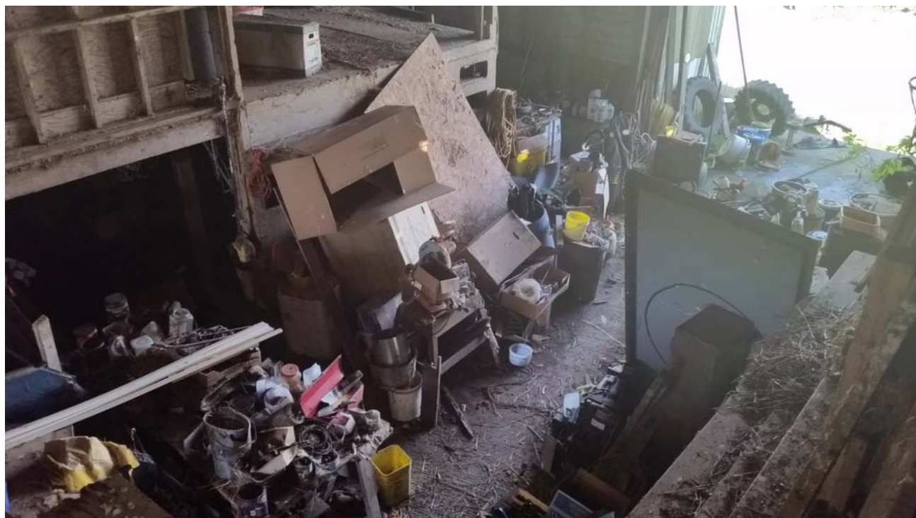
PHOTO 6: View of east breezeway from loft.
