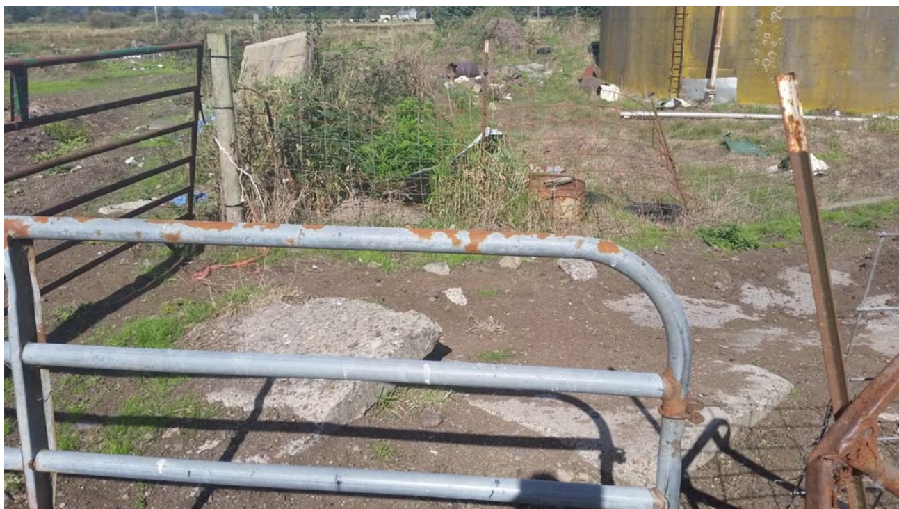
PHOTO 14: Fill material south of farm buildings and manure tank. Concrete pieces were from demolition of loading dock at a local dairy.
