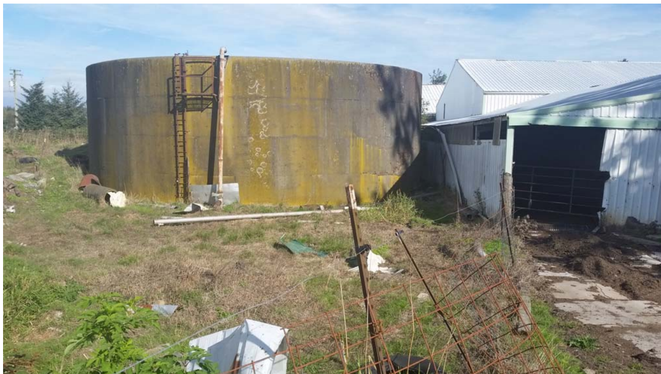
PHOTO 13: Above-ground liquid manure tank on southwest corner of loafing shed.
