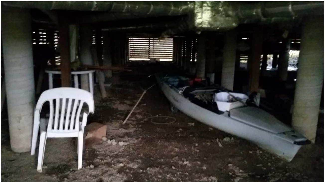
PHOTO 8: Crawlspace under house.
