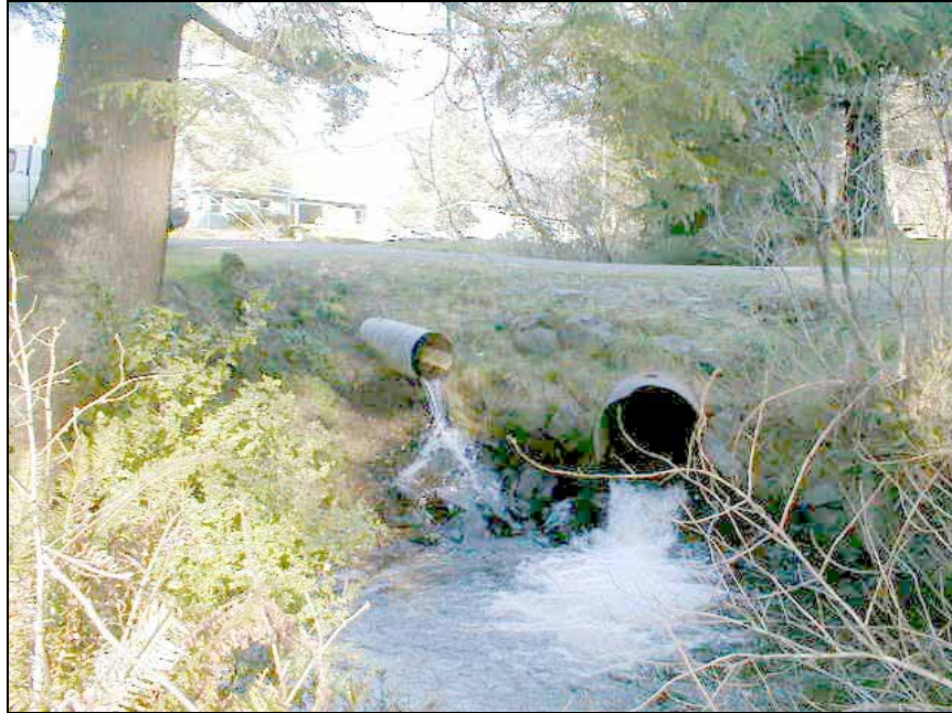
Figure 15 - Perched Culvert Example
