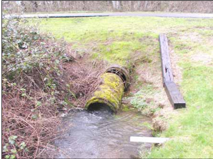
Figure 13 - Broken Pipes Example
