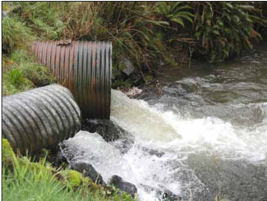
Figure 16 - Perched Culvert Example
