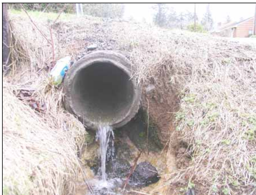
Figure 18 - Scoured Culvert Outlet
