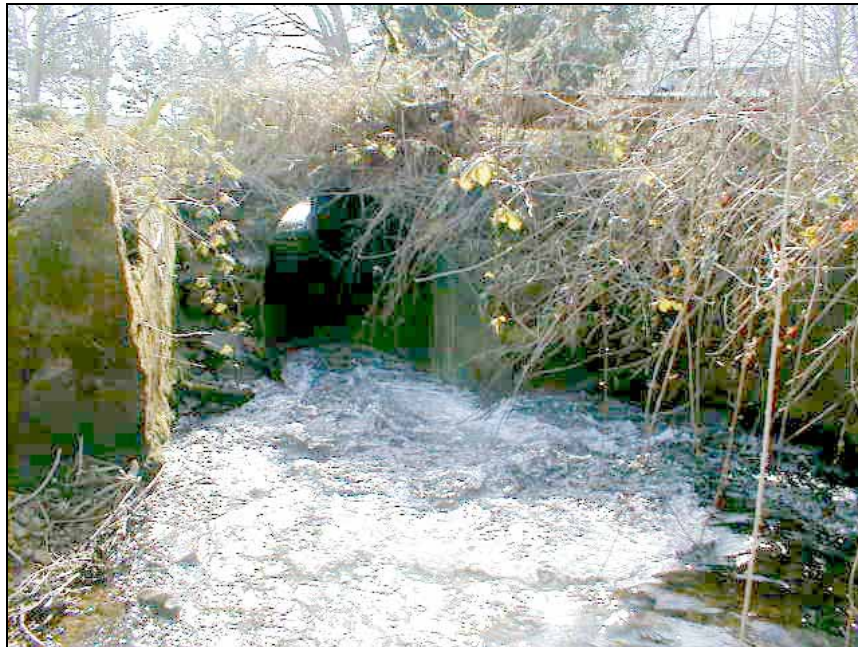
Figure 14 - Scoured Bottom Culvert
