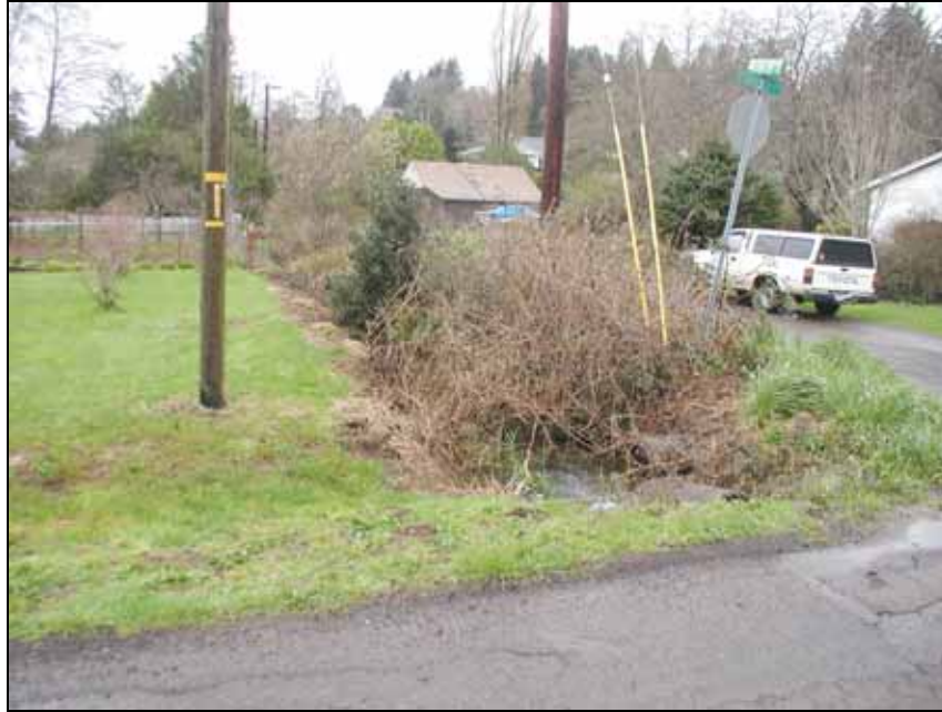
Figure 19 - Overgrown Ditch Example
