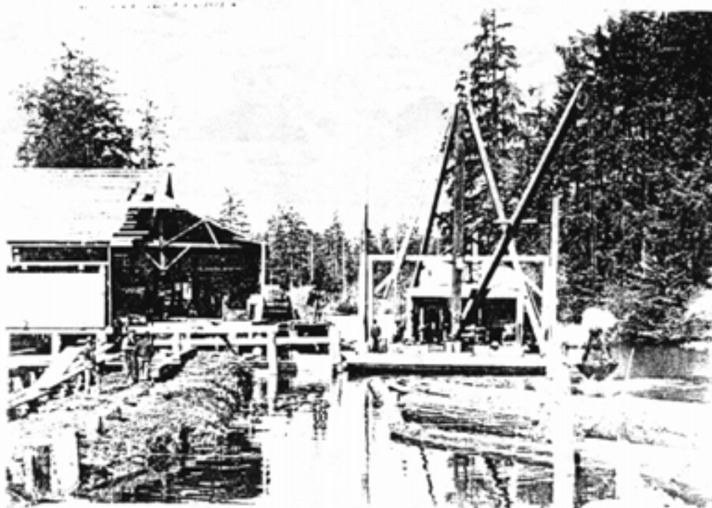
Dredging in Hoquarten Slough, circa 1905
