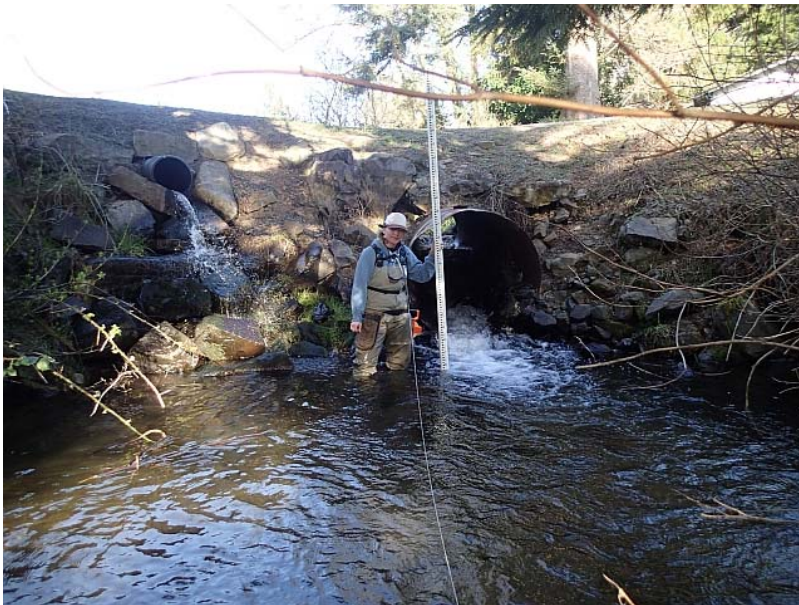
Figure 18: Crossing 575 (7th St.). The plastic culvert fed by the 7th Street drainage ditch can be seen on the left bank of the crossing fill. Downstream scour pool is 3' at deepest point.
