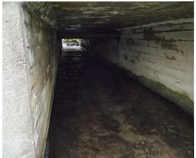
Figure 27: Exposed sewer main inside Crossing 578. Visible near top of box culvert
