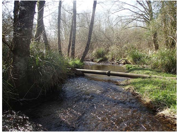
Figure 26: Exposed sewer main crossing Patterson Creek (Reach 1)
