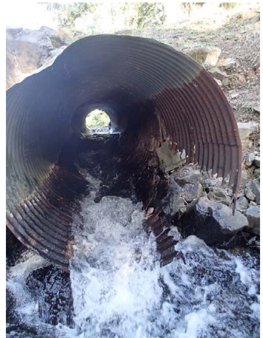
Figure 19: Outlet of Crossing 575, showing complete pipe failure. Scour has eroded below the pipe, which now projects above the pool below. Total perch height is 12" from water surface to outlet of pipe.
