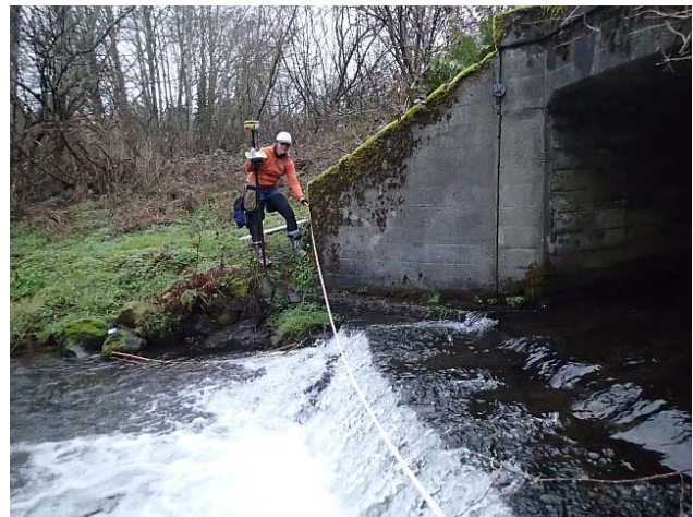
Figure 1: Locating culverts with GPS-RTK survey unit. Survey staff use a combination of methods including tapes and level rods.
