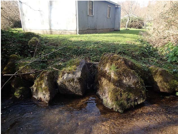
Figure 11: This reach currently has multiple revetments and stream bank protections to prevent erosion both above and below confluence with Jacoby Creek.
