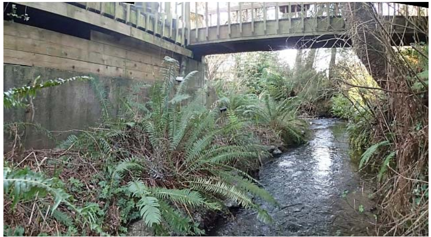
Figure 15: Residential development extends to the average high flow water level in Reach 5, limiting the potential to aggrade the channel as an approach to removing the fish passage barrier at the existing fish ladder, upstream approximately 200 feet.
