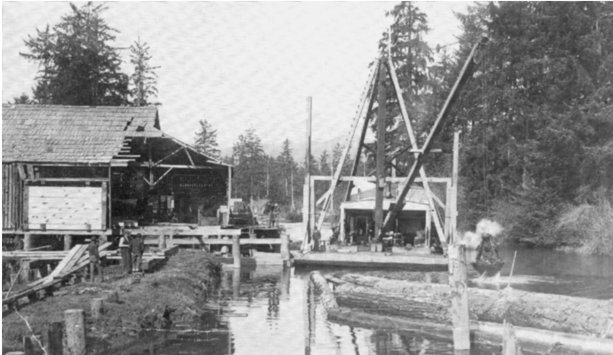
Government dredge at work in Hoquarten Slough near the town sawmill. (c. 1900). Photo Courtesy of Tillamook County Pioneer Museum.
