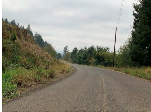
Image 18: Eastern 0.5 to 1.5 miles in fair condition
