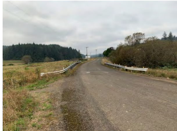
Image 20: Beaver Creek bridge on Eckloff Road, facing west
